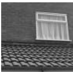
Type E Cavitraye installed in a wall showing where a perp weepvent is fitted to the tray.
